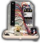
End Tower Box
